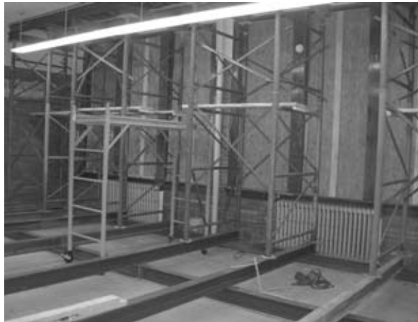
A kindergarten classroom under renovation.
